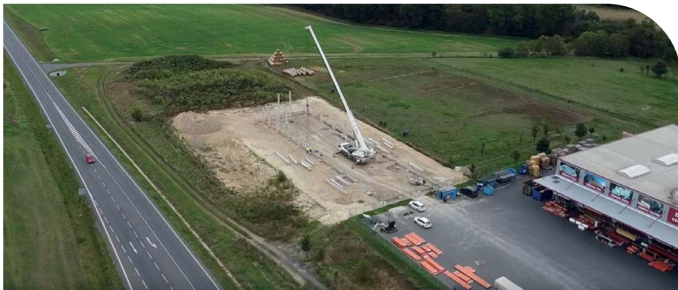
September 2025: Piling for the reinforced concrete 'barn' in the neighbourhood of COMAX ROOFS
